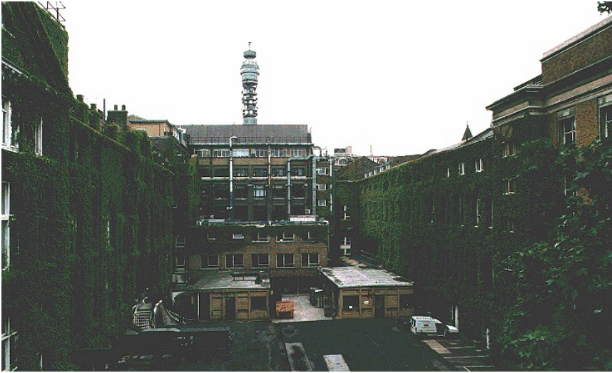
The “circular car park” base site
