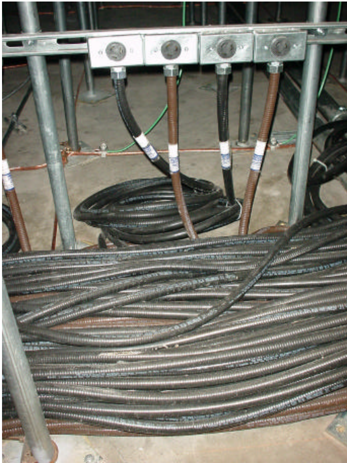
Under Floor Space
