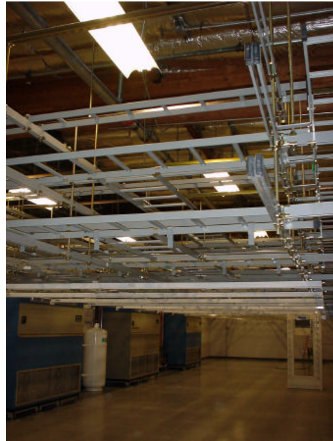
Overhead Cable Tray
