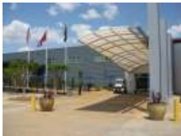
QTS Metro Data Center (Atlanta); 970k sqft and Tulip Data City in Bangalore, India (“largest in Asia”)
