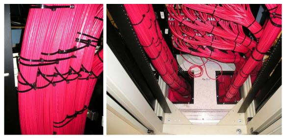
Figure 3: Pictures of the cabling tested.
