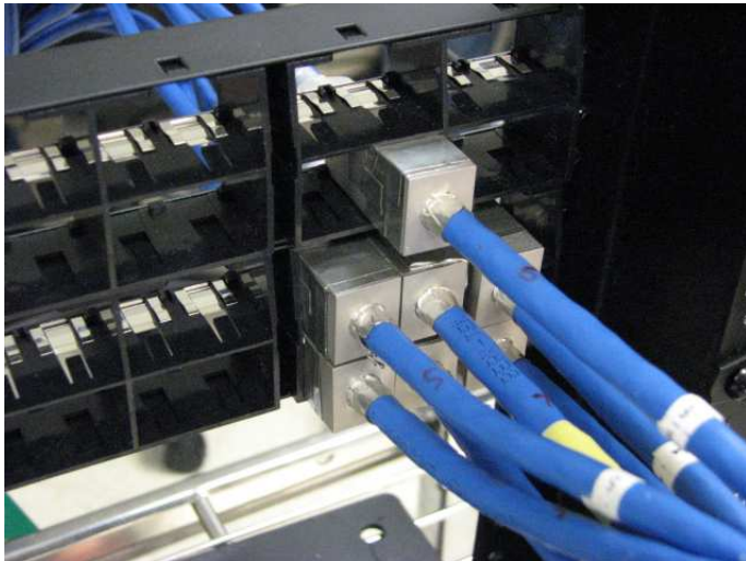
S-RJ45 Horizontal cable side of patch panel
