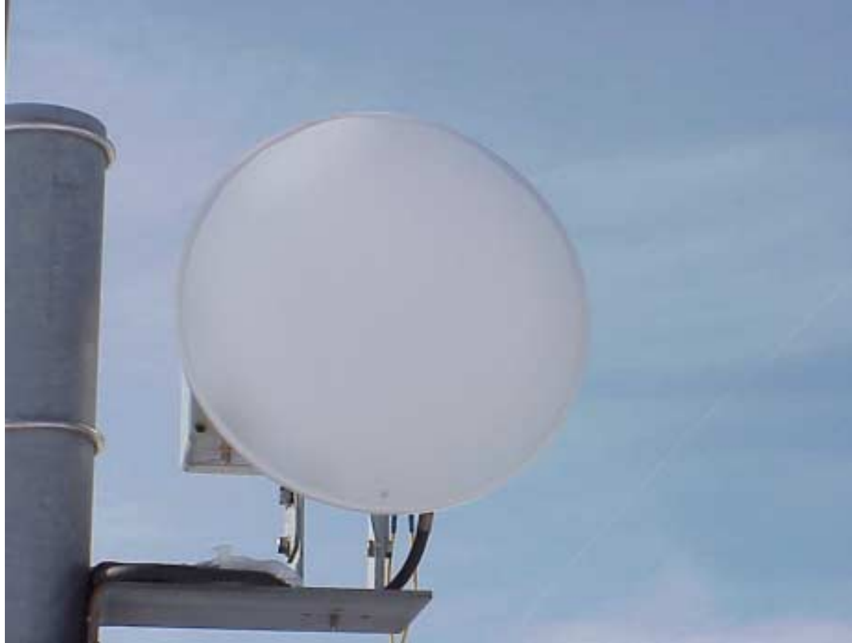
Half Mile Solution with Parabolic Antenna
